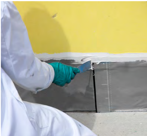
Example of bridging from below grade water proofing to Air Barrier using Dow Corning ® 758 Silicone Weather Barrier Sealant
