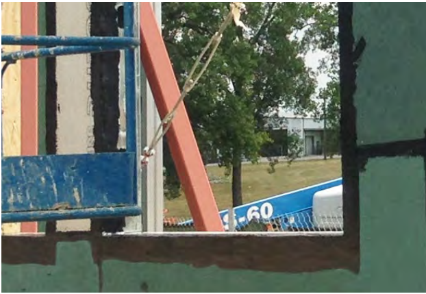
Example of flashing at window opening
