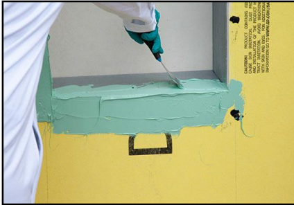
Figure 1: Application of Dow Corning 778 Liquid Flashing.
