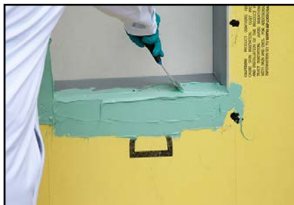
Figure 1: Application of DOWSIL 778 Silicone Liquid Flashing.
