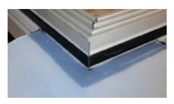
DOWSIL™ Silicone Transition System is a flexible, durable suite of silicone materials designed to help you create flexible transitions between various types of air and water barriers and the curtainwall, storefront, or window
